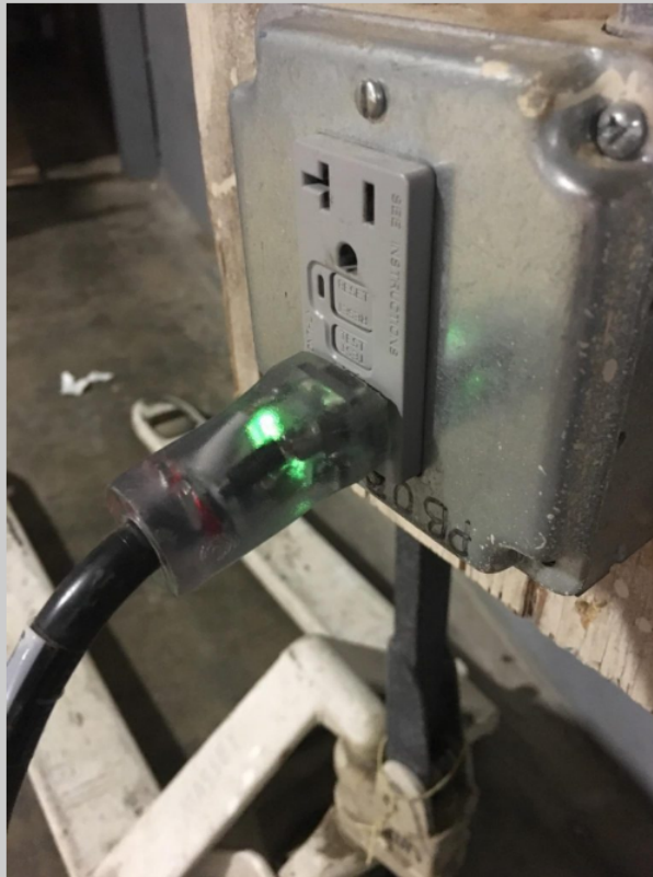
Ground Light Indicator showing that the OUTLET and cord are grounded.
